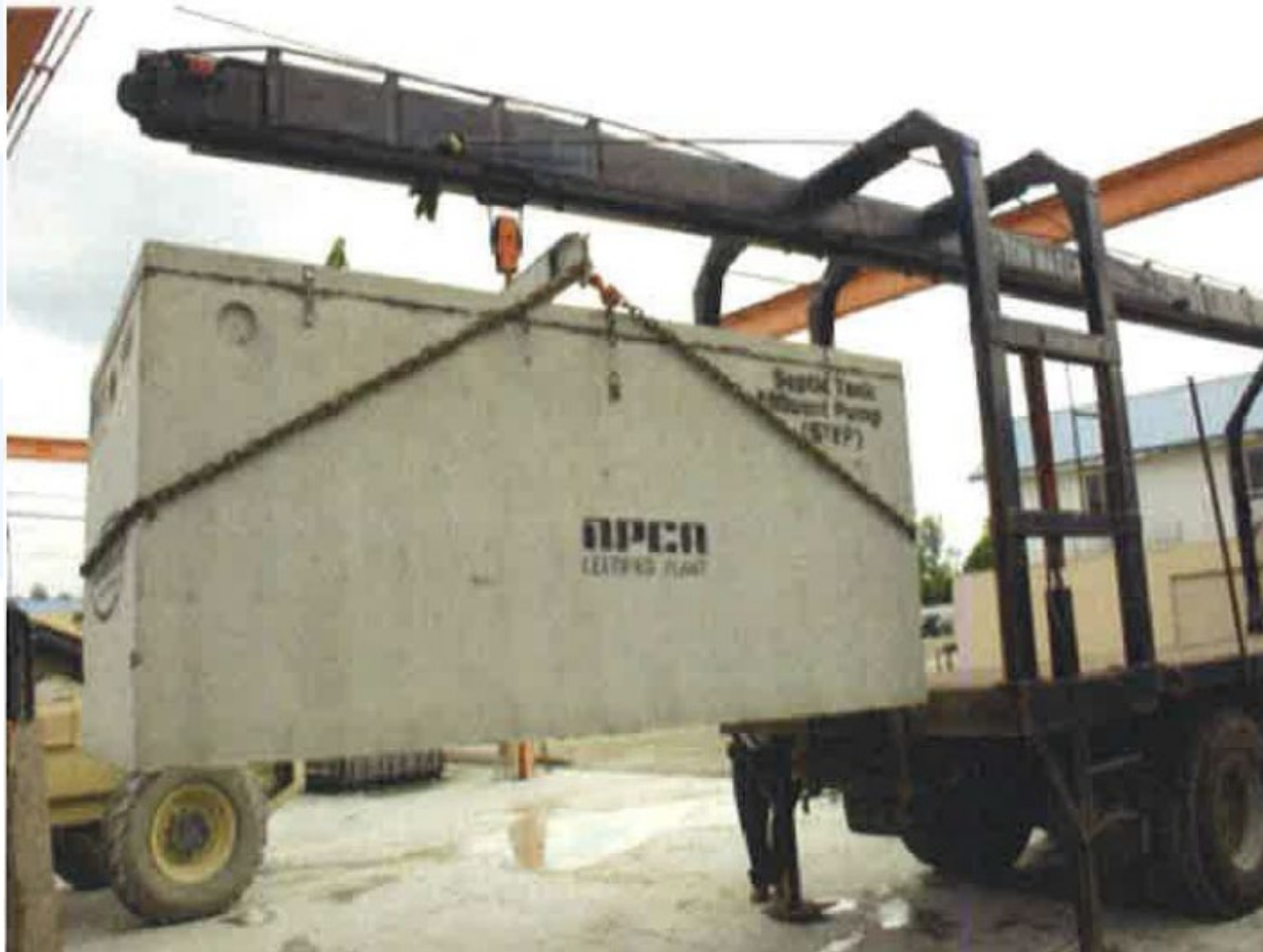
Photo 3: Septic Tank Delivery Rig
